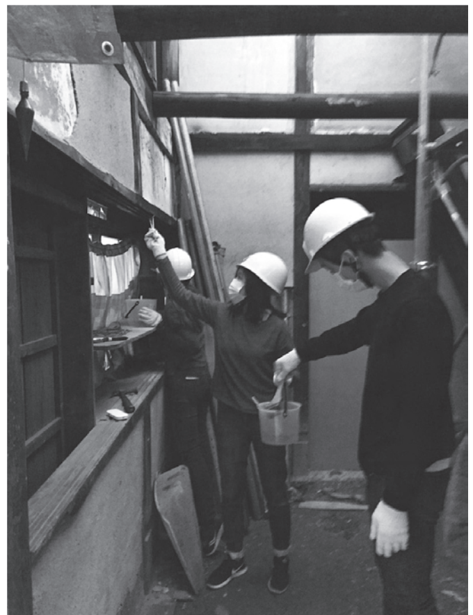
Students learning how to renovate traditional Japanese wood frame buildings.
